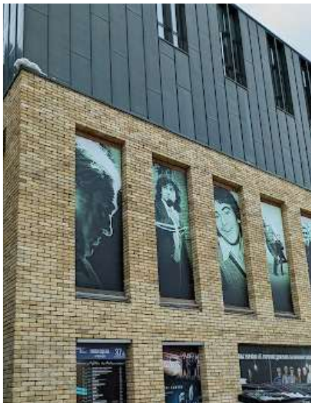
figure 6. Reused brick facade on the Theatre on Podil by Drozdov&Partners. Kyiv, Ukraine, Dec 2023
