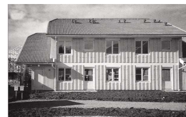
New detached housing built from salvaged precast panels at Gothenburg, Sweden (Image: Geiselmann, 1991)
