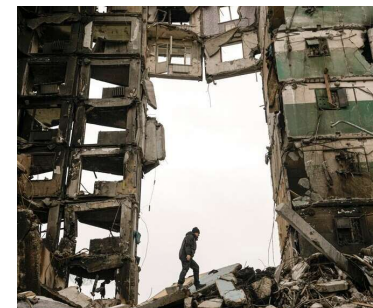
Collapsed Khrushchevka Building made of precast concrete panels in Ukraine (Web image 5)
