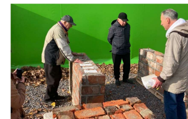
Testing the construction of insulated cavity walls built of reclaimed bricks (Image Daniel Wyss)
