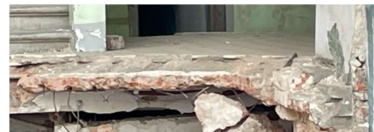
An old slab in Kharkiv, made of concrete and old bricks
