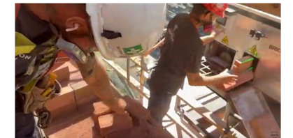
In-Situ brick trimming in Canada Image: Youtube
