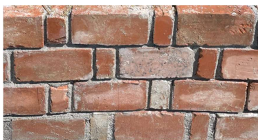
Rowlock Bond with reclaimed bricks and waste-based insulation (Balkans, SDC, HEKS, VoRAE, Skat) | D. Wyss
